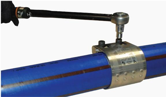
6. Tighten the hex socket head bolts until the set torque is achieved in each bolt. For the straight couplers, which have two bolts on a double width shell, tighten the bolts alternately and evenly until set torque is achieved in each bolt. The pipe will relax after the set torque is achieved, so after a minute or more, retighten the bolts to the set torque. Repeat until less than a quarter turn is needed to reach the set torque\*.
