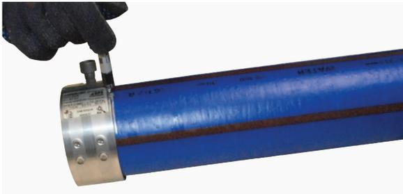
5. Push the repair coupler inserts into the repair piece and position into the cut section.
