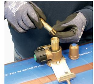
*NB. The liner must be installed and stops any water from penetrating the pipe layers. Failure to fit the liner will result in the pipe de-laminating and will void the approval.*
