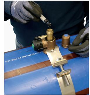
6. Ensure the cutter is fitted with the liner before installing it in the ferrule body. The cutter shall be turned down flush with the top of the body before fitting the ferrule cap. Make sure the small seal is placed correctly in the cap.
