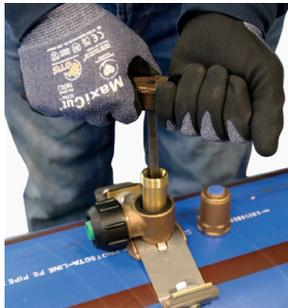
5. The pre-cutter will remove the swarf generated by the drilling. Check for any additional swarf that hasn't been removed fully before moving onto the next step.
