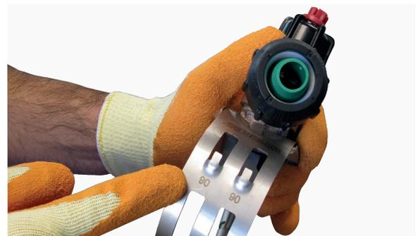
2. Unhitch the lower part of the ferrule understrap from the tabs on the upper part of the strap. Leaving the bolt in place, fit the ferrule squarely around the main, re-attach the understrap to the appropriate tabs.
