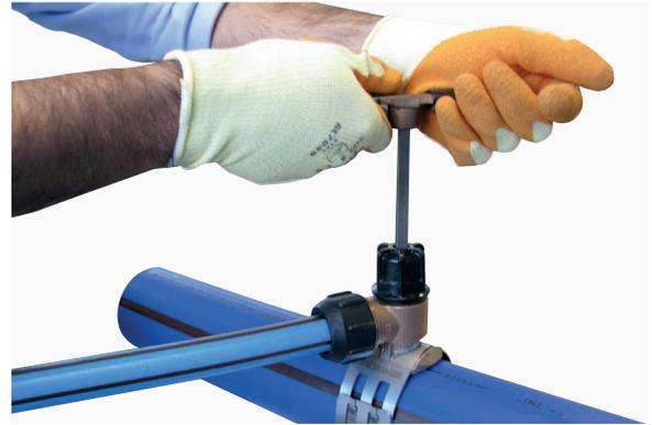
6. Withdraw the cutter all the way up to the top of the stem, employing a final counter-clockwise torque of 12-14Nm to ensure a good seal. Some leakage through the plughole is normal before the cutter has been fully unscrewed. Replace the plug.
