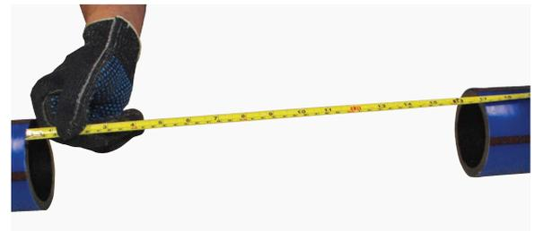
3. Fit the half shells to the ends of the cut out section and mark the penetration depths.
