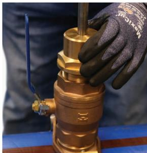
4. Attach the 110V power drill to the drill stem and apply slight pressure whilst drilling the main until there is no resistance (main wall drilled).
