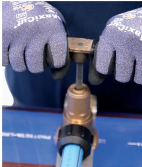
*NB. You should feel growing resistance before the cutter turns easily and then stops. It is normal to get slight discharge of water during this operation.*
