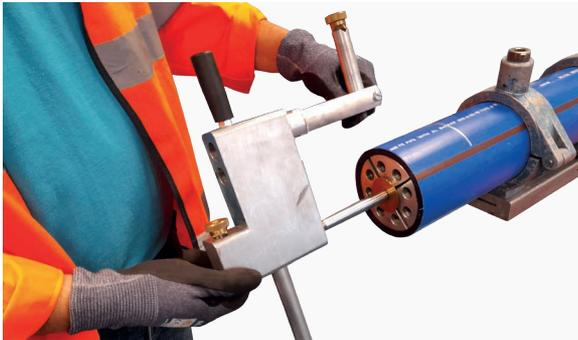
6. Slide the body of the Protecta-Line surprep scraper onto the mandrel, depress the release button and position the cutter close to the edge of the pipe.
