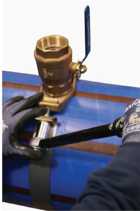
*NB: For main sizes 315mm and 355mm, apply a torque of 40Nm - 44Nm.*
