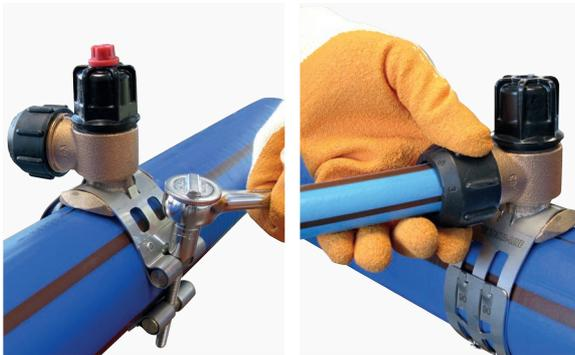
4. Fit the Protecta-Line service pipe into the compression fitting on the outlet, as described in the instructions on page 37. After aligning the outlet to the desired position, tighten the securing collar and compression fitting. **Test T and connections prior to drilling.**
