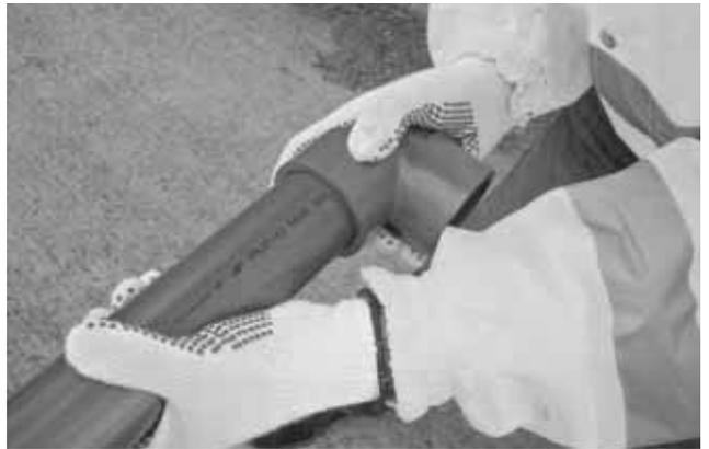
10. Wipe off excess cement from the outside of the joint.
