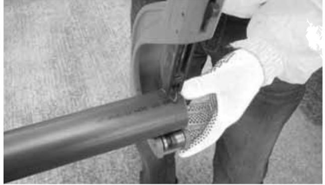
8. Install Centra-guide support at pipe's end. Distance between the fitting and support should not exceed  $1\frac{1}{2}$  metres. Install additional supports if required.
