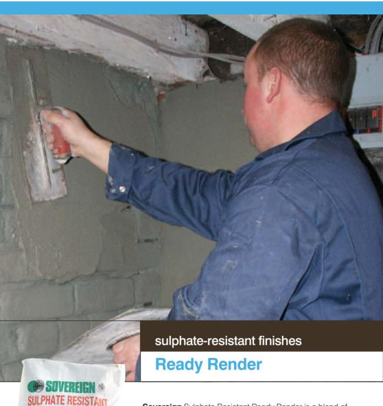
**Sovereign** Sulphate Resistant Ready Render is a blend of cement, fine sands and lime combined with special additives that minimise 'water demand' whilst also improving workability and adhesion. The dry-blended mix has been developed for both internal or external application onto most traditional masonry backgrounds, such as brickwork and blocks.
