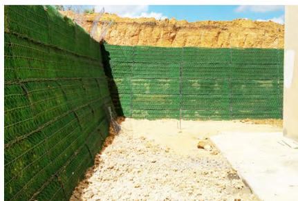
Photo 5 - Coating of the face of containments in soil reinforced with MacMat® 10.1
