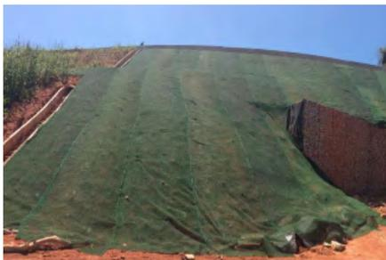
Photo 1 - Slope cladding above a retaining wall in gabions with MacMat® R3
