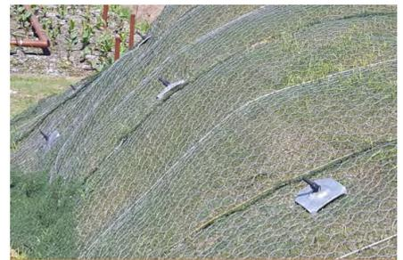
Photo 3 - Coating the face of a stapled soil with MacMat® HS
