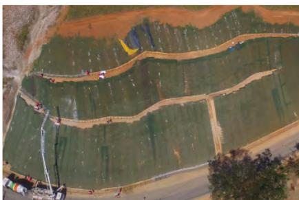
Photo 4 - Coating of the face of a soil stapled with MacMat® HS or MacMat® R1
