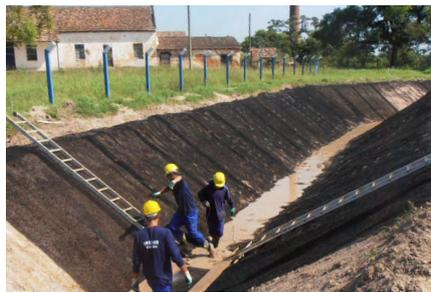
Photo 2 - Stormwater drainage channel coating with MacMat® 10.1
