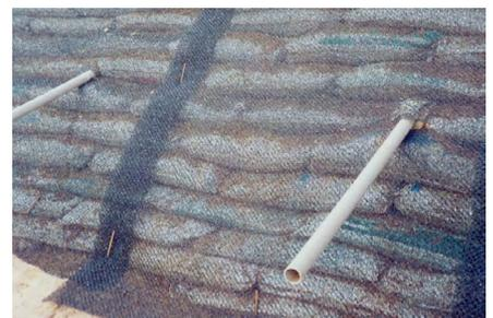
Photo 6 - Coating of the face of an erosion recovery with rip-rap with MacMat® 10.1
