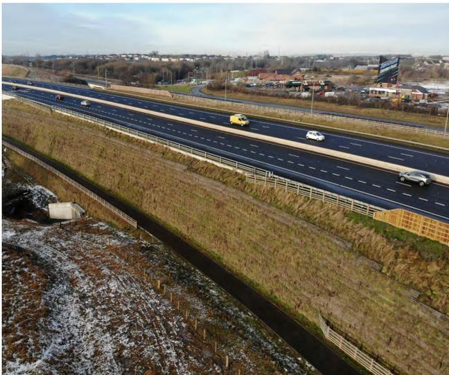
**Green Terramesh®** is an environmentally friendly modular system. When used with ParaGrid® or ParaDrain®, suitable site-won materials can often be used as structural backfill to the reinforced soil slope.
