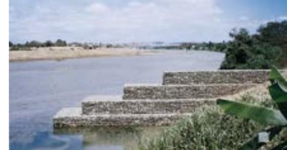
As groynes reduce the littoral longitudinal transport they are normally implemented with a beach nourishment scheme, with the overall objective of reducing shoreline erosion. Groyne works can also be combined with submerged offshore breakwaters.
