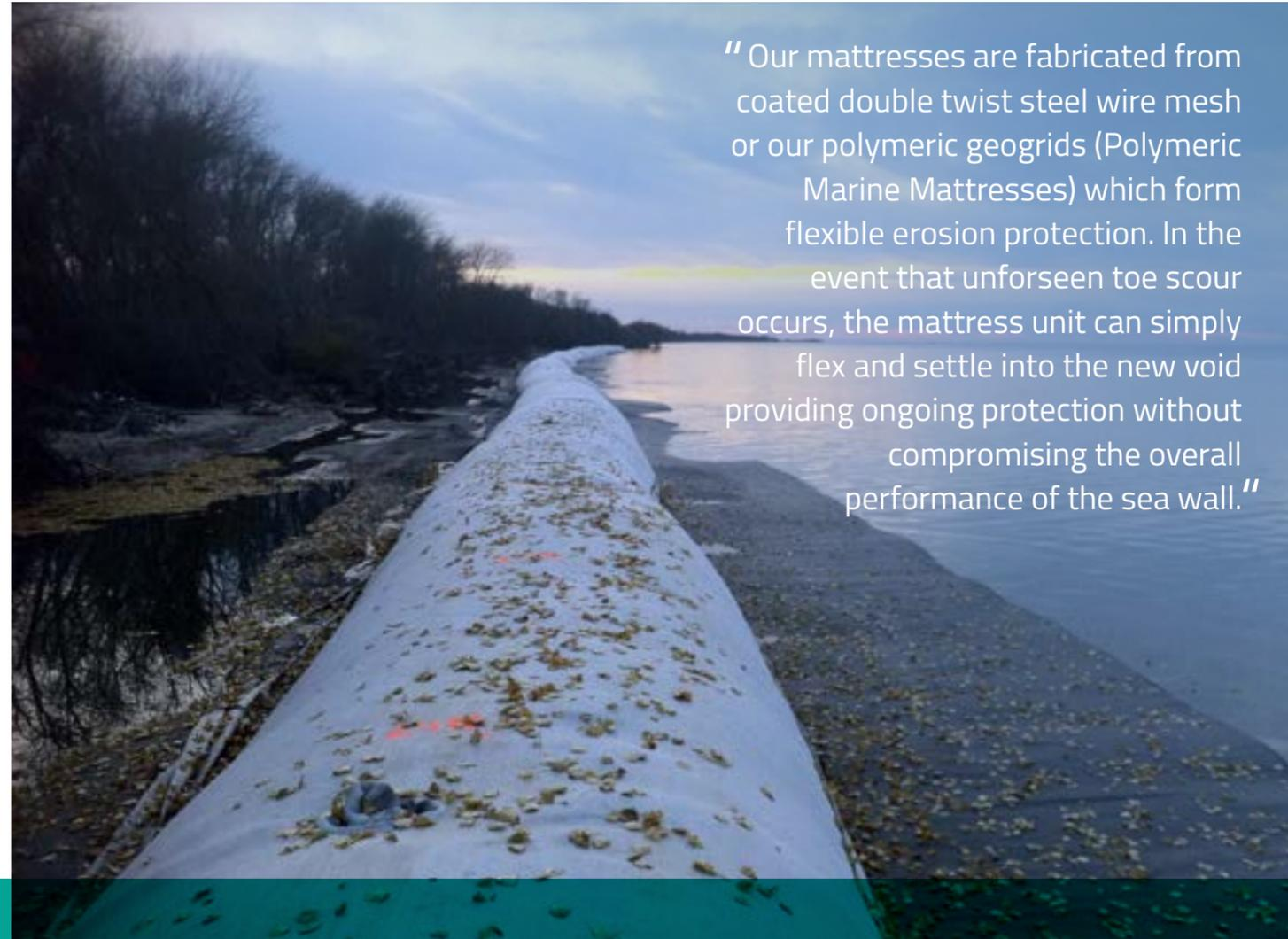
“ Our mattresses are fabricated from coated double twist steel wire mesh or our polymeric geogrids (Polymeric Marine Mattresses) which form flexible erosion protection. In the event that unforeseen toe scour occurs, the mattress unit can simply flex and settle into the new void providing ongoing protection without compromising the overall performance of the sea wall.”
