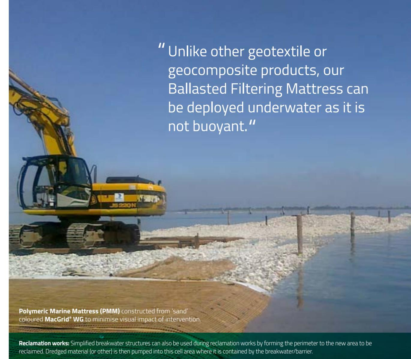
**Polymeric Marine Mattress (PMM)** constructed from 'sand' coloured **MacGrid® WG** to minimise visual impact of intervention.
