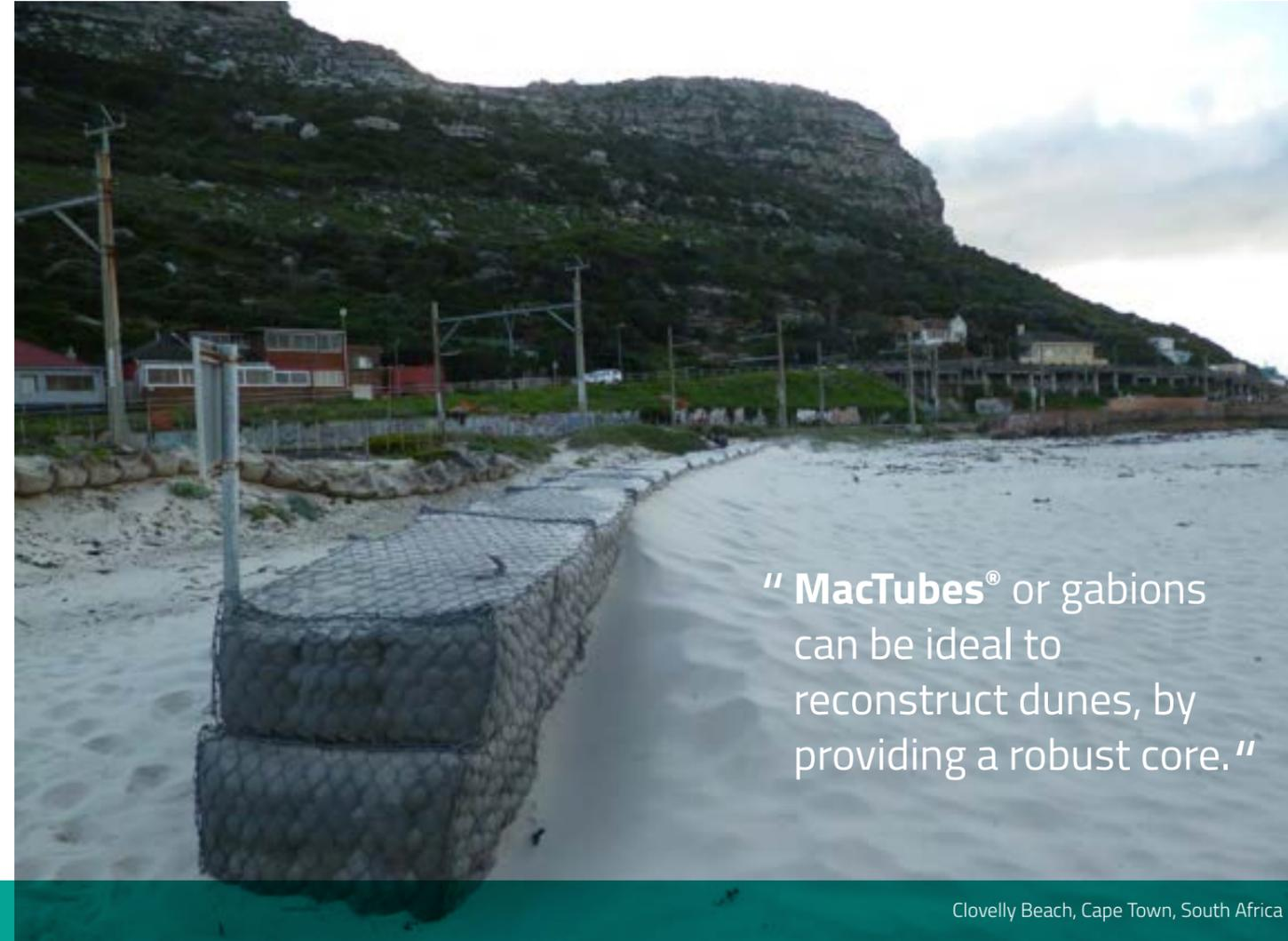
“ MacTubes® or gabions can be ideal to reconstruct dunes, by providing a robust core.”
