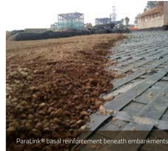
ParaLink® basal reinforcement beneath embankments
