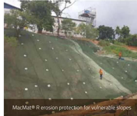
MacMat® R erosion protection for vulnerable slopes
