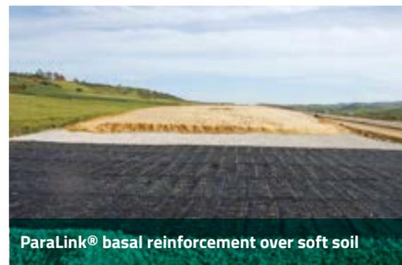
ParaLink® basal reinforcement over soft soil
