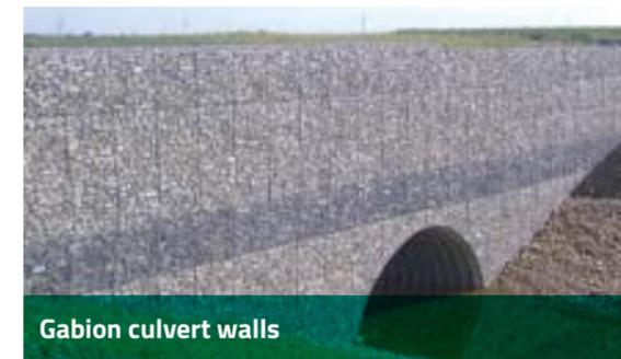
Gabion culvert walls
