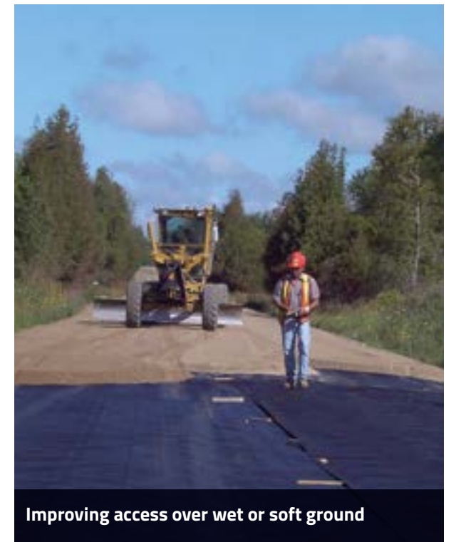
Reinforcing pavements over peat
