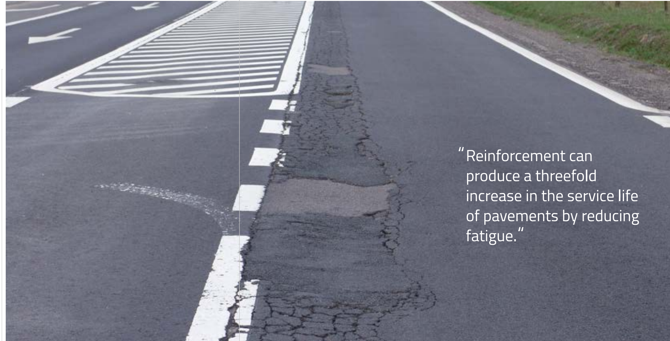
Reinforcing pavements over peat
