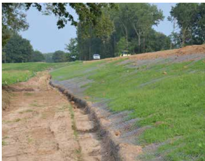
Anti-burrowing mesh installed on highway embankment
