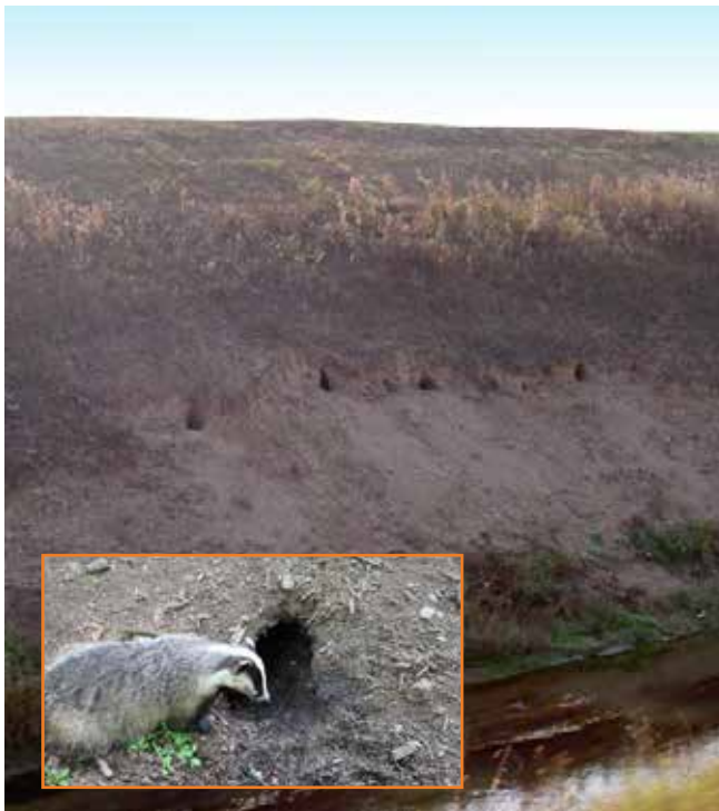
Mammal burrow damage to slope causing vegetation loss and instability
