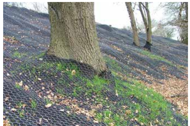
DT mesh flexibility enables variable slope profile and obstacles to be accommodated easily
