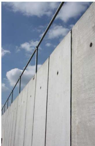
has the basic ability to act as a retaining structure in general applications such as ground walling, perimeter boundaries and changes in levels, mainly where constraints such as access and time are paramount. The Rockwall retaining units can be cast in to new concrete slabs or anchored down to new or existing concrete foundations.
