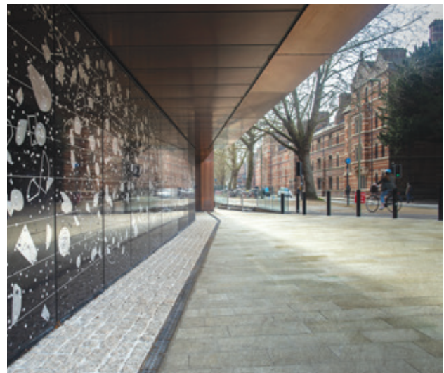
ACO MultiDrain MD with ductile iron grating, Beecroft physics department, Oxford
