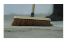
Sweep the area to be painted so that it is clean and free of loose material. New concrete should be left for at least 28 days.
