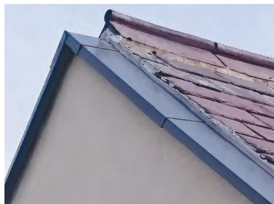
Sealant must be applied to the inside edge of the WEC 771 OVERTRIM.
