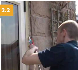
The door can now be fully sealed with silicone and cleaned.
