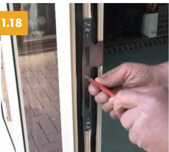
Traffic door keep adjustment is achieved by using the screws, which simply need to be loosened, in order to give inward and outward adjustment. Once the keep is in the correct position carefully retighten the screws.
