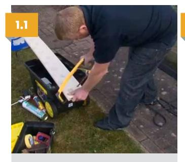
Measure and cut the base cill to size. Glue the cill end caps on to the cill.
