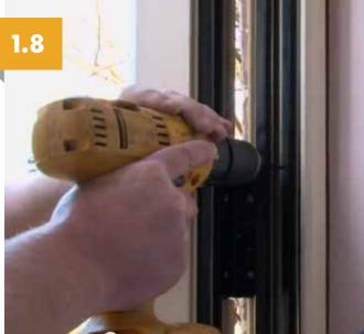
Fixings in the jambs should be fitted through the centre line of the euro groove. The suitable fixings for this installation are available from all Eurocell building plastics depots.
