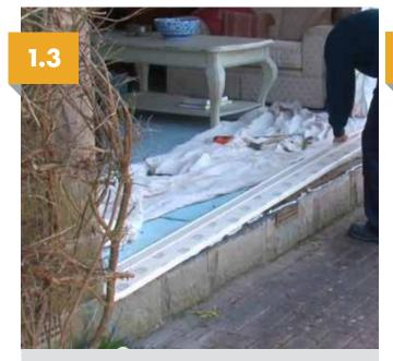
Apply a generous bead of silicone across the bottom of the aperture to sit the base cill on and fix the cill to the aperture ensuring that it is level.
