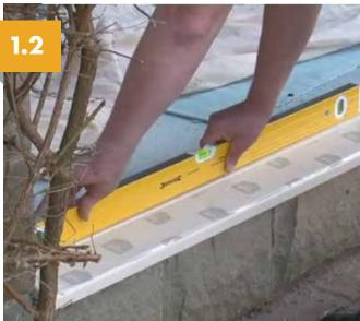
Offer the base cill into the opening, check the cill is level across its overall length (maximum deviation is 3mm).
