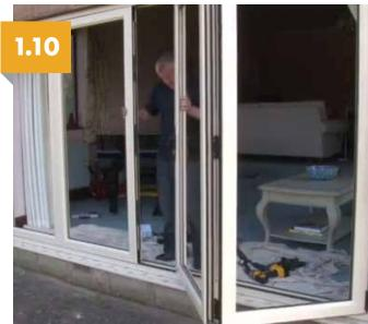
Check that the sashes operate correctly before the glazing begins.
