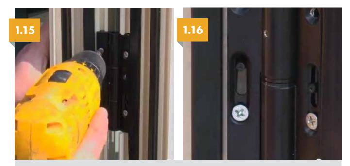
Hinge adjustment is achieved by loosening off the 2 screws on each leaf and then sliding the adjuster peg to suit, once the lateral adjustment has been made please ensure to carefully tighten the screws. (5mm lateral & 2mm height adjustment available per hinge).
