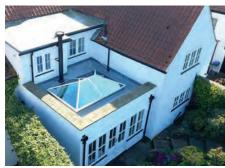
Korniche 'All Aluminium' roof lanterns are based upon a popular wooden-framed design prominent in the Victorian-era. Thanks to its die-cast aluminium components and patented method of fixings, it can span up to 3m x 2.5m for a single piece of glass per side, or up to a maximum roof space of 6m x 4m with intermediate rafters – the perfect solution for large area glazing.
