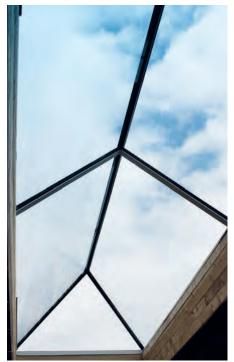
Thermalight roof lanterns have a contemporary and unique design that utilises the latest state-of-the-art technology in structural silicone glazing, creating a totally frameless product with one of the slimmest sightlines on the market.
