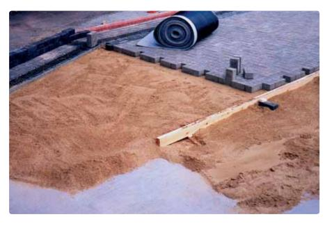
waterproofing membrane is required below the block paving (e.g. roof top car parks or tanked SuDS pavements).
