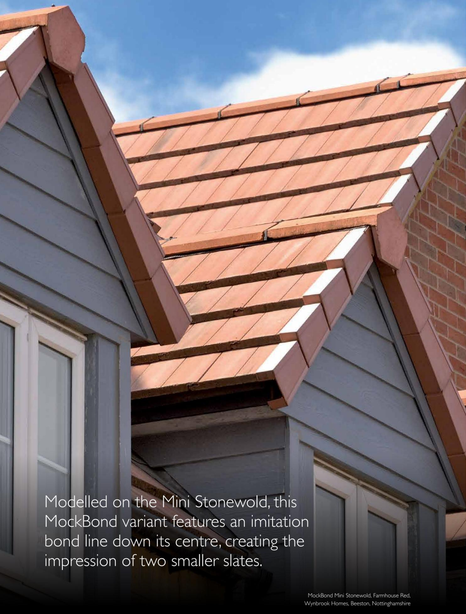
Modelled on the Mini Stonewold, this MockBond variant features an imitation bond line down its centre, creating the impression of two smaller slates.
