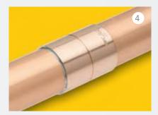
**4.** Allow the joint to cool without disturbance. Clean the joint generally, wiping off any external flux residues. This will prevent unsightly stains or (in extreme cases) corrosion of pipework. Flush out the pipework.
