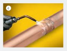
**5.** Apply the filler rod to the mouth of the fitting, allowing the brazing alloy to melt and flow into the annular gap.
