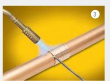
**3.** Apply solder to the mouth of the fitting. When the correct temperature has been reached the solder will flow freely and be drawn into the joint. Briefly reapply the blowtorch and wipe off any excess solder.
