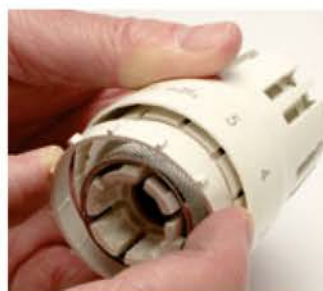
2. When engaged, the tool is twisted and pulled down to remove the inner ring. The head is lifted and rotated so that the plastic arrow above the thermal ring aligns with the required temperature setting number.
