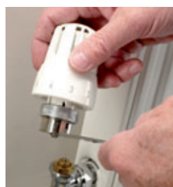
2. The thermal ring is screwed into the threaded adaptor at the base of the tool. This compresses the clips on the TRV head and allows the ring to pop off. The ring becomes more difficult to turn as the compression increases and it is sometimes necessary to use grips to increase leverage.
