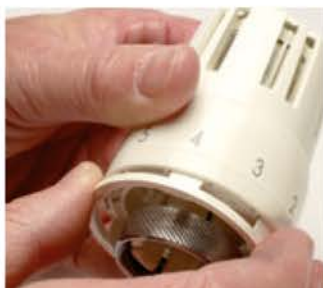
1. The lugs on the removal tool should be inserted into the grooves on the inner ring of the TRV head.
