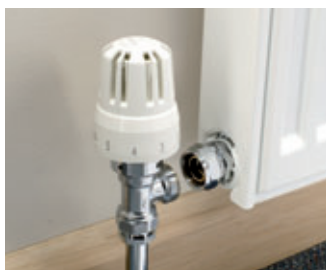
2. The new radiator valve is attached to the pipe work and the tailpiece extended and connected to the valve.
