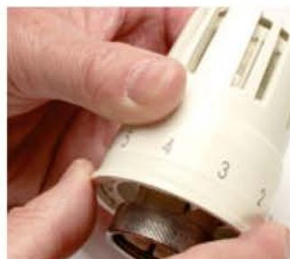
1. The lugs on the removal tool should be inserted into the grooves on the inner ring of the TRV head.
