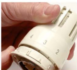
2. When engaged, the tool is twisted and pulled down to remove the inner ring. The head is lifted and rotated so that the plastic arrow above the thermal ring aligns with the required temperature setting number.
