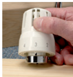
5. The TRV head is pressed onto the anti-theft thermal ring until they snap together.
