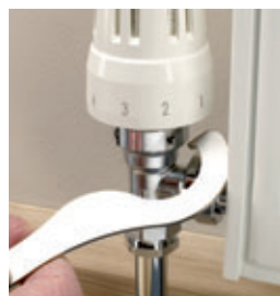
6. The standard thermal ring can be unscrewed and removed from the tool and the 'C' end of the tool used to tighten the ring onto the valve.
