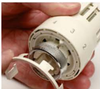
1. The lugs on the removal tool should be inserted into the grooves on the inner ring of the TRV head.
