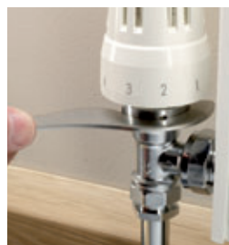
6. The standard thermal ring can be unscrewed and removed from the tool and the 'C' end of the tool used to tighten the ring onto the valve.
