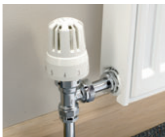
2. The new radiator valve is attached to the pipe work and the tailpiece extended and connected to the valve.
