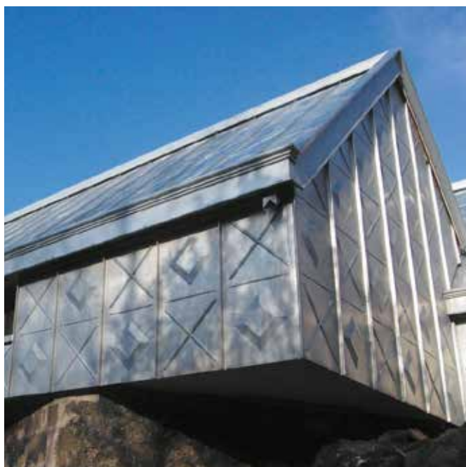
After crimping (double crimped standing seam)
