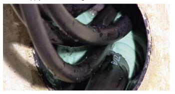
3. Slightly elevating the services, inject about 100 mm of sealant, slowly pulling back ensuring that all voids are filled
