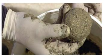
6. When fully mixed, form a ball or mortar. Add more water as required until the ball is stable and does not fall apart
