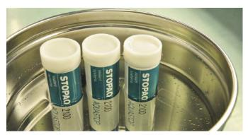
1. Preheat the cartridges to 30°C. This makes the sealant much easier to apply via the mastic gun
