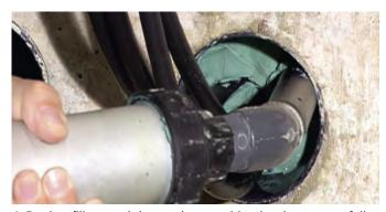
4. Further fill around the services, pushing hard to ensure full compaction and to within 50 mm of the wall
