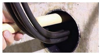
2. Insert a piece of foam to act as a back-stop, pushing into the duct with a stick so that it is 150 mm in from the wall surface
