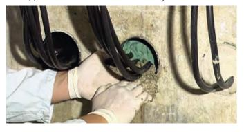
7. Push the mortar tightly into the sleeve to the wall surface to fill the remaining 50 mm of depth with mortar
