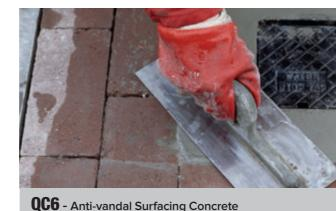
Ideal for the surface reinstatement of 'picture frames' or fillets and around access covers and for general repairs in
