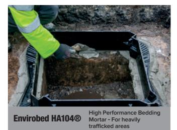
The environmentally friendly alternative to resin-based materials. Ideal for bedding ironwork, gullies and linear drainage.
