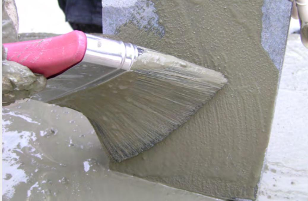
*Failed paving is costly. The addition of a slurry primer to a paved construction is essential to guarantee a bond strength compliant with BS 7533.*
