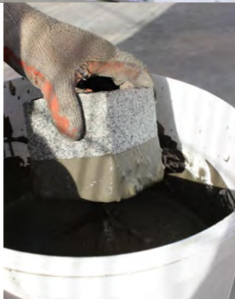
The addition of a priming layer between the paving element and bedding mortar yields an extremely high bond strength which prevents this type of failure. This increases the life expectancy of your paved area and reduces its ongoing maintenance and potential litigation costs.
