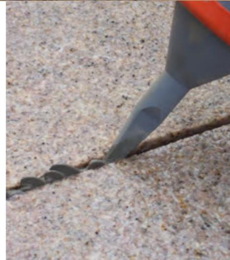
*UltraScape's cempoint gun injected mortar is perfect for those smaller areas which can be difficult to grout. Fast and easy to apply, with no wastage, it neatly and directly fills the paving joint.*
