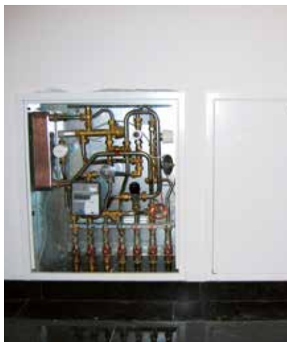
Recess mounting in a floor and kitchen.
