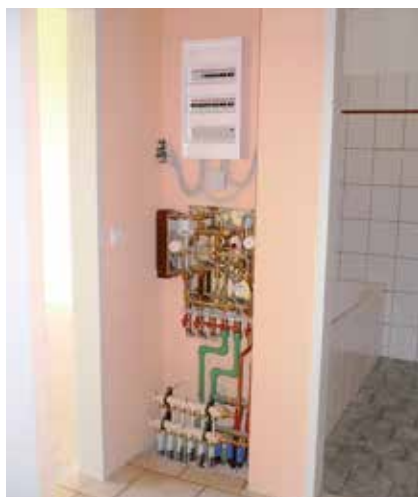
A flat station mounted in a shaft or cupboard.
