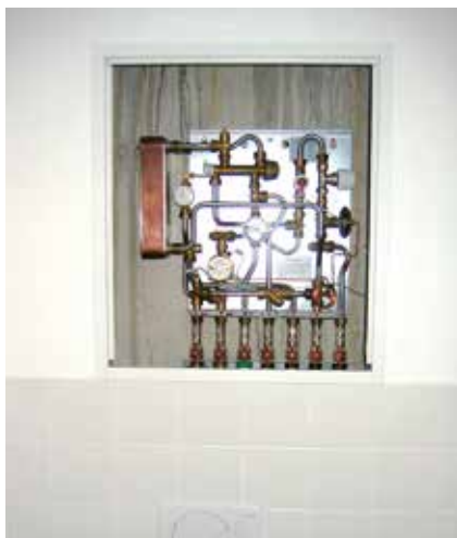
Recess mounted flat station in a bathroom shaft.
