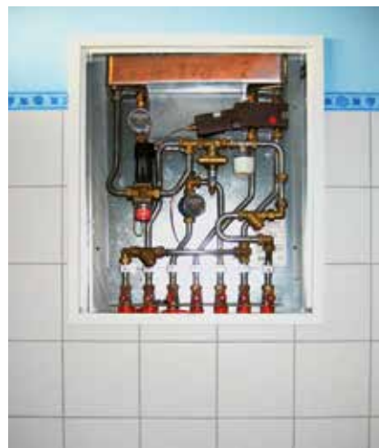
Recess mounted flat station in a bathroom.
