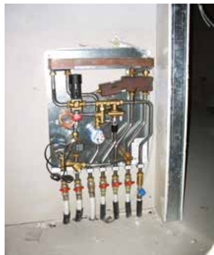
On-wall mounting of a flat station.
