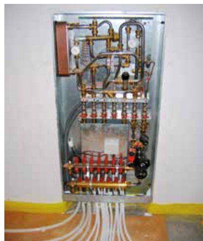
Recess mounting of a flat station with a floor heating distribution unit.
