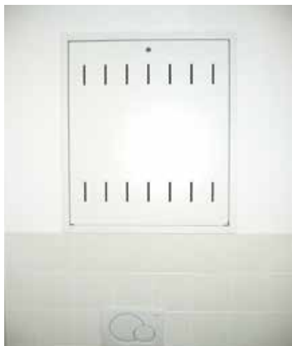
Flat station with cover, recess mounted in a bathroom shaft.
