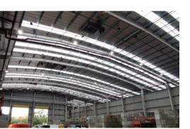
weights can provide a variety of safety levels. Filon rooflights are supplied as natural translucent GRP but coloured opaque and tinted sheets can also be manufactured.
