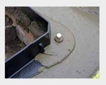
Continue to mix and pour the mortar until it covers the base and the flange of the frame to a level of 20mm above the flange ensuring 100mm remains to the surface of the carriageway. This is indicated by the height on the nylon cap which sits on the flange.
