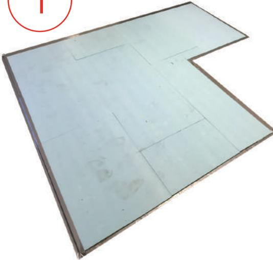
**1.** Before installation, the subfloor must be clean, dry, level and all protrusions removed. Lay the Gaia-XPS insulation, ensuring the whole floor is covered. To prevent movement, fasten with tape, DO NOT use any type of spray adhesive to stick the insulation down.
