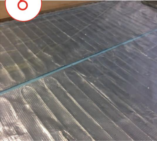
**6.** The floor finish can now be installed. Always install the floor finish in accordance with the manufacturers requirements. Ensure the flooring is suitable for use with underfloor heating and has been acclimatised to the room following manufacturers guidelines before installing. Leave room for expansion around the edge of the room if the flooring manufacturer states this is required.
