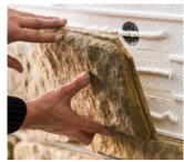
Apply stone slips between ribs ensuring each piece is firmly seated with full contact to panel.
