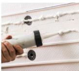
6. Apply a generous bead of high grab adhesive ¾ of the way up each standard course, ensuring the fastener head is covered. For a double or triple course sized slip, use 2 or 3 beads of adhesive respectively.
