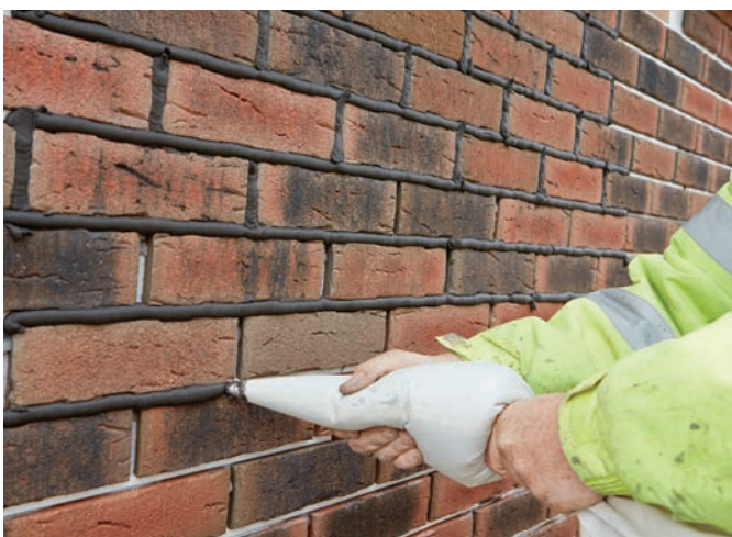
Applying mortar
