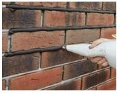
**3.** Specially formulated mortar is then piped into the brick joints.
