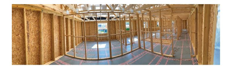
SMARTPLY SURE STEP is a tongue and groove OSB/3 panel with a high-performance and durable coating for improved performance during the construction phase of projects. It is an airtight panel, certified by PHI in Germany, for use in floor or decking as part of the airtightness layer of low energy and passiv buildings.
