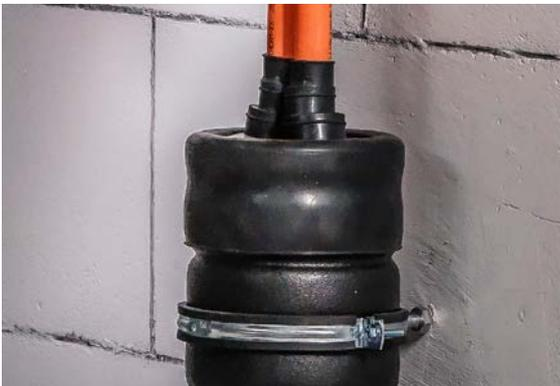
Fig. 05-23 Closing pipe with rubber end cap
