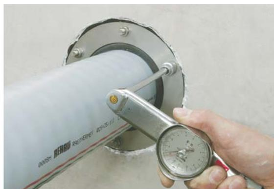
Fig. 05-12 Installation using a torque wrench
