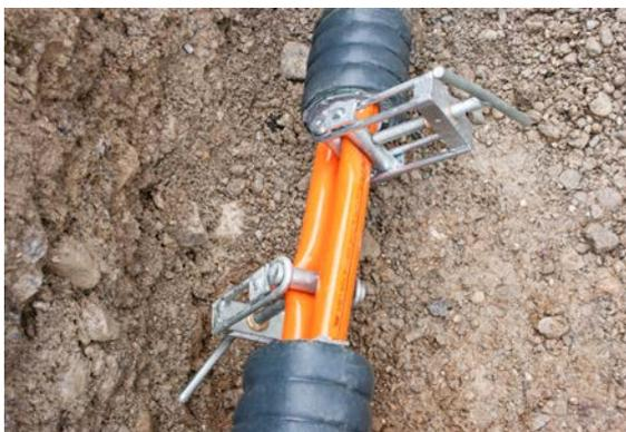
Fig. 07-32 Squeezing off DUO carrier pipes
