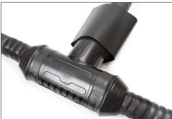
Fig. 04-24 Fitting the heat-shrink T-shroud
