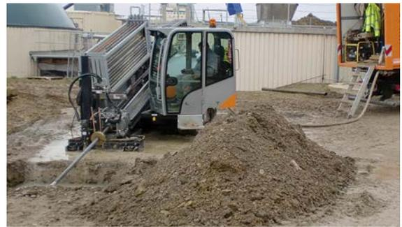
Fig. 07-10 Installation with horizontal directional drilling device
