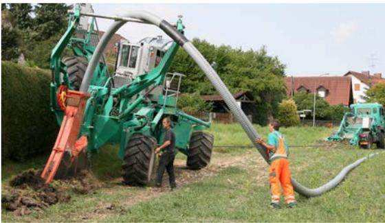
Fig. 07-8 Installation with mole ploughing machine
