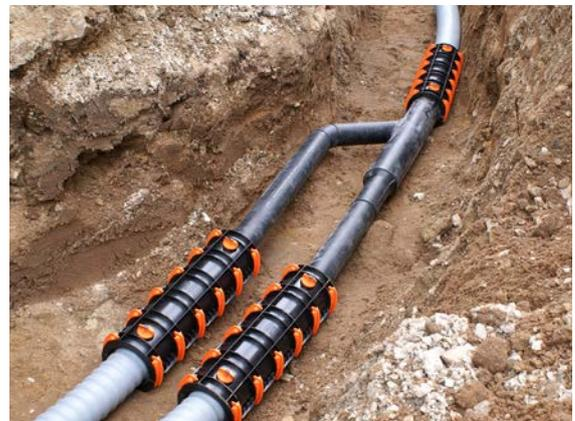
Fig. 04-34 Y-pipe installation in practice
