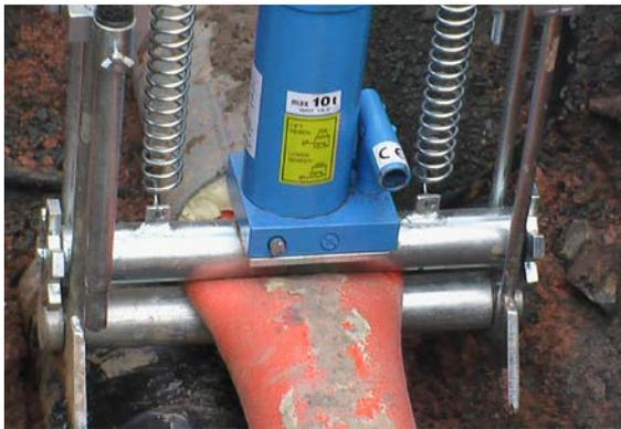
Fig. 07-31 Squeezing off UNO carrier pipes
