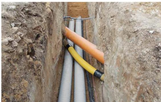
Fig. 07-22 Passing beneath crossing lines
